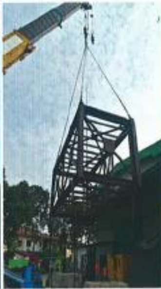
LOAD TEST WORK IN PROGRESS & HOLDING TIME : 10 MINUTES.
